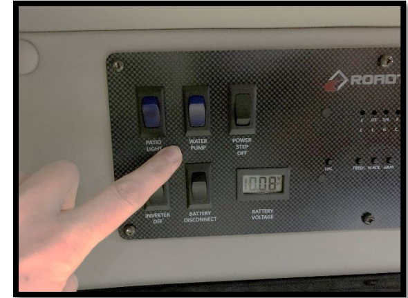
Picture 42.2 Water Pump Switch
