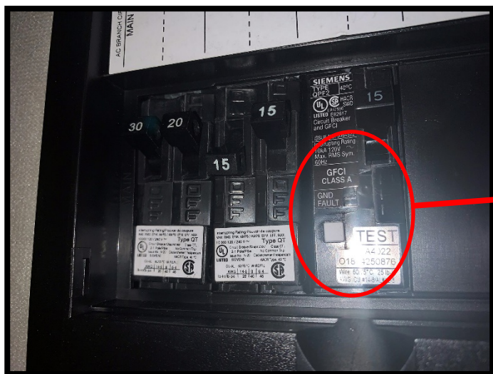
GFCI located on the fuse panel above the driver's seat
