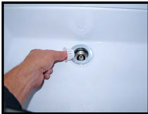
Picture 26.2 Shower drain
