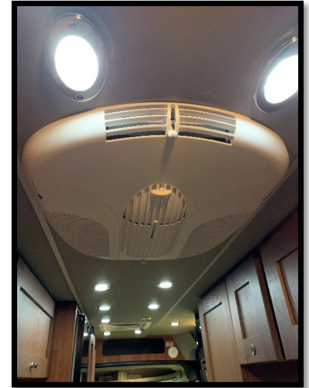
Picture 36.3 Roof-mount air conditioner
