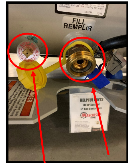
Propane bleed valve and propane fill valve
