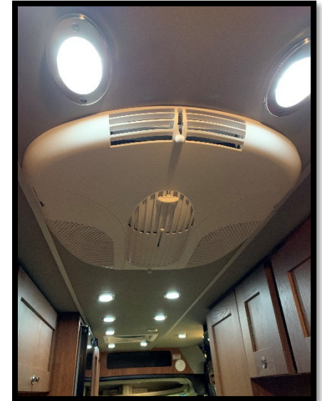
Picture 36.3 Roof-mount air conditioner
