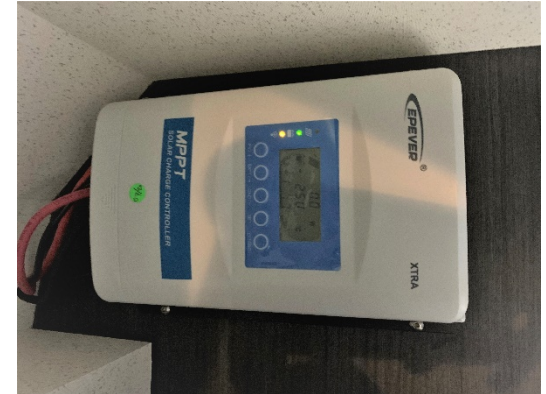
Picture 38.1 Solar charge controller
