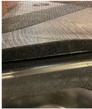
Picture 32.2 Hook and loop fastener for bottom edge of screen
