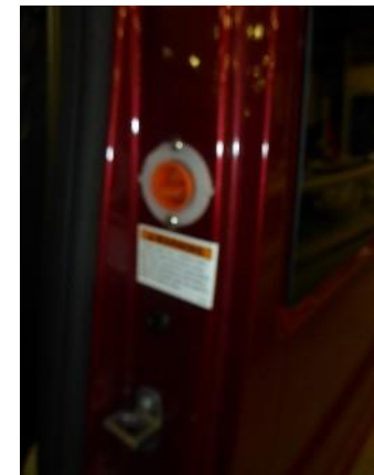
Fresh water tank fill location
