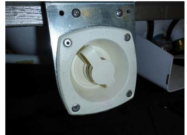
Built-in pressure regulator
