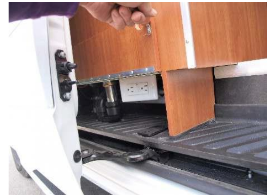
The city water valve is behind this access panel to the left of the side door opening
