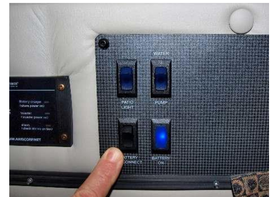
Battery disconnect switch
