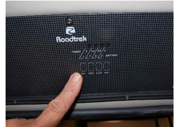
Tank and battery level indicators
