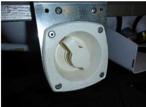
Built in pressure regulator
