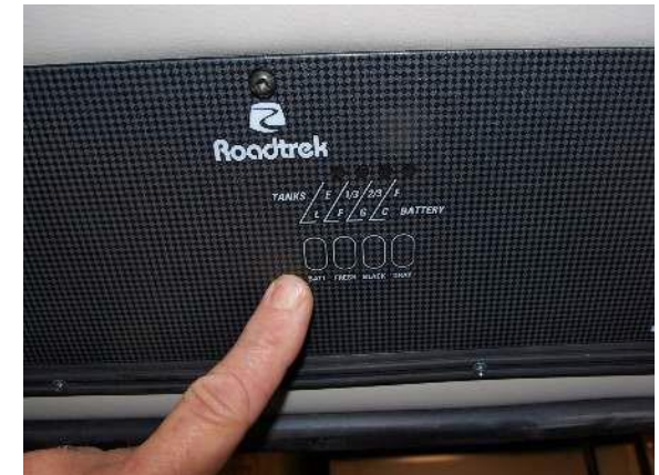
Tank and battery level indicators
