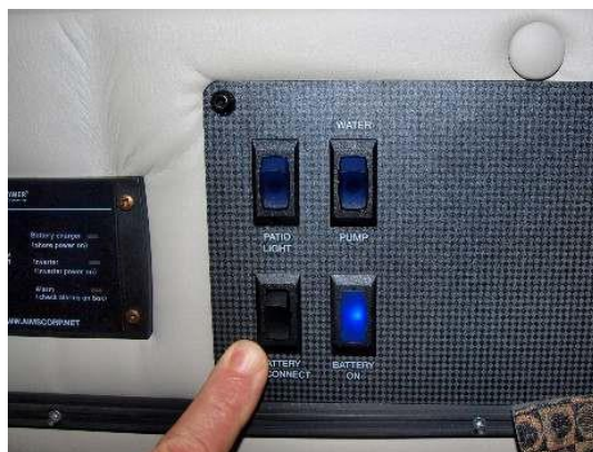
Battery disconnect switch
