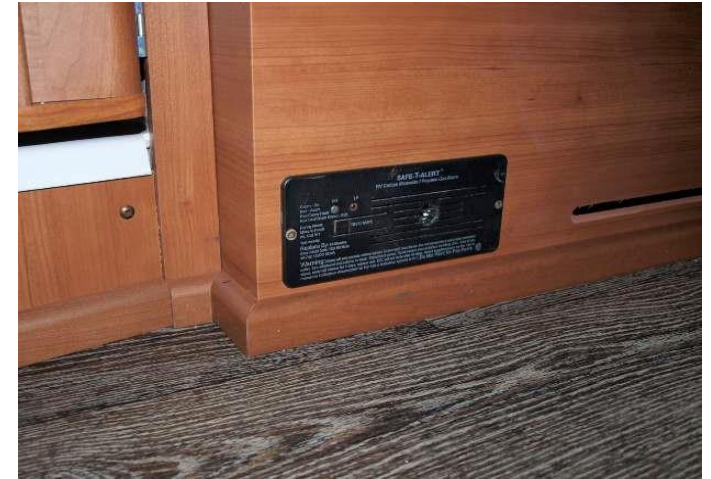
Propane and Carbon Monoxide alarm
