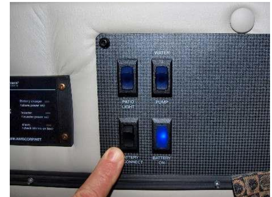
Battery disconnect switch
