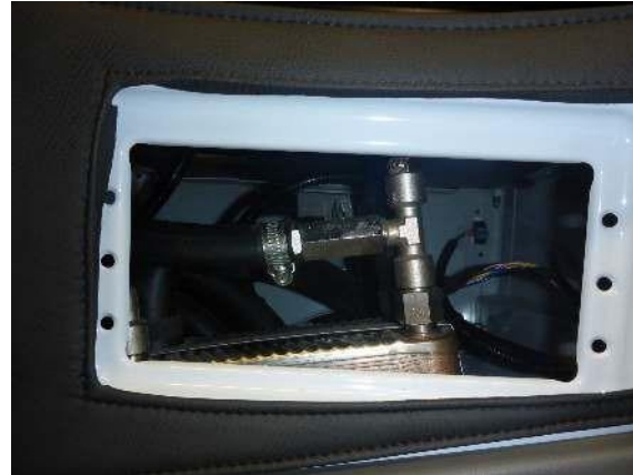
The heat exchanger valve. Valve open (as shown) allows the heat exchange to take place.
