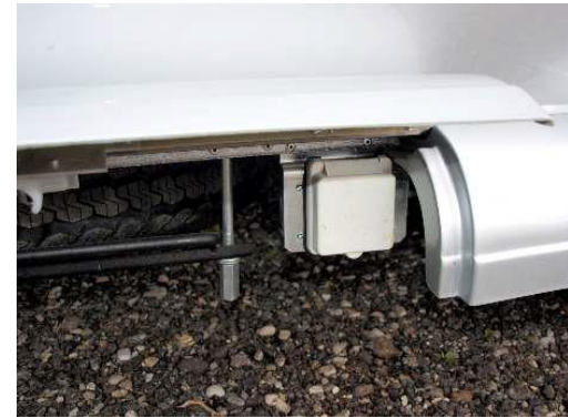
Shore Power connection point
