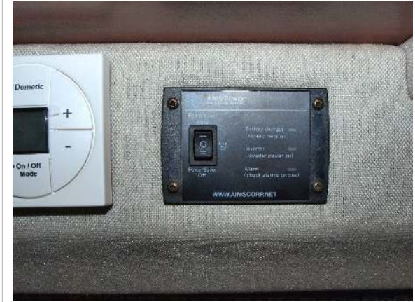
Inverter switch for optional 2500 watt inverter
