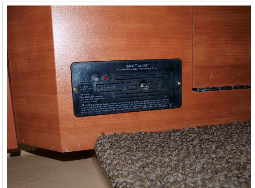
Propane and CO alarm
