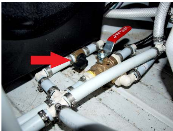
Tank isolator valve in open position (black plastic handle pointed horizontally). This valve is located inside the hot water heater enclosure, at the base of the large black speaker on the back wall.
