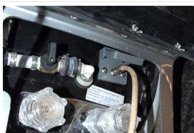
TV cable connected
