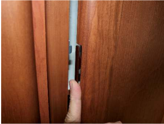
Hidden latch along edge of cabinet door
