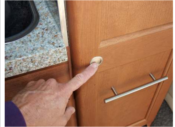
Locked pushbutton latch on cabinet door
