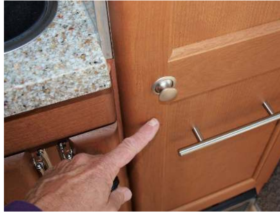
Pushbutton latch on cabinet door
