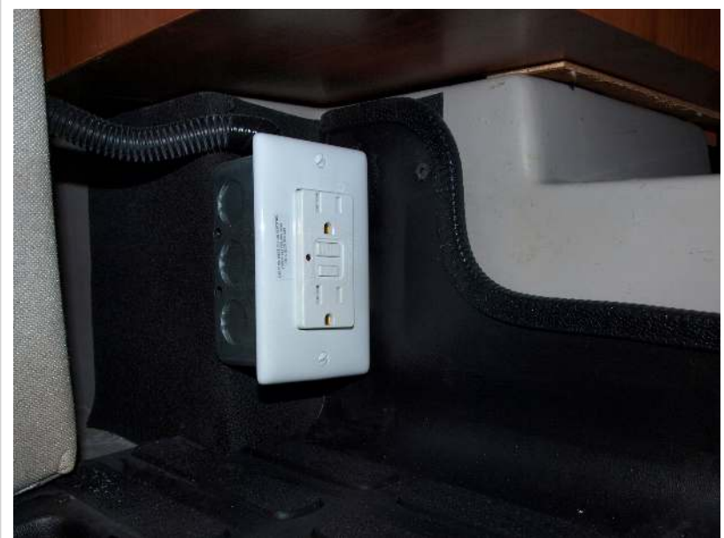
GFCI outlet under rear passenger side seat
