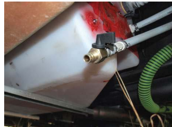
Freshwater tank drain valve
