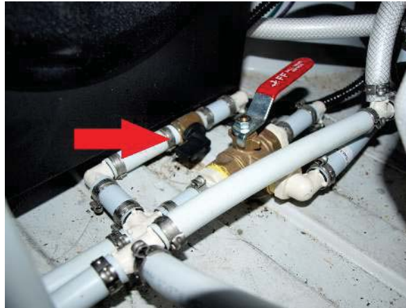
Tank isolator valve in open position (black handle pointed horizontally).
