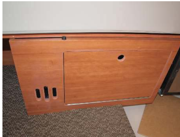
Water heater enclosure
