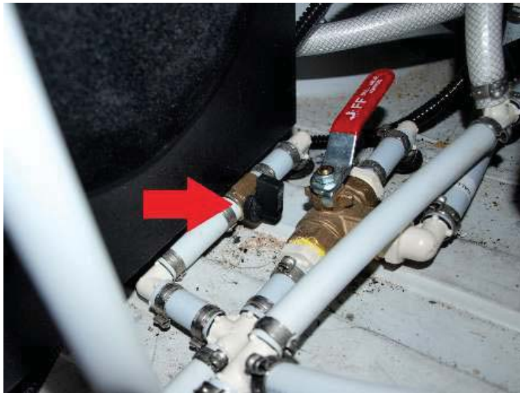
Tank isolator valve in closed position (black plastic handle pointed up). This valve is located inside the hot water heater enclosure, at the base of the large black speaker on the back wall.
