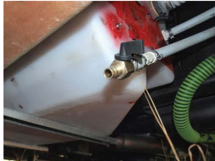
Exterior tank drain, under driver's door step
