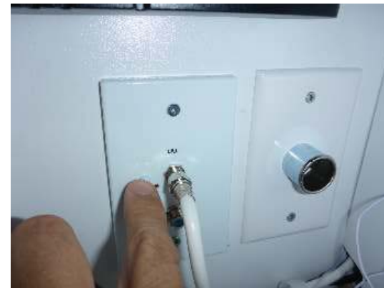
antenna/cable AB switch selected for cable (bottom button)
