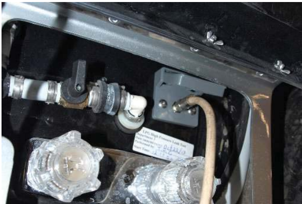
TV cable connected
