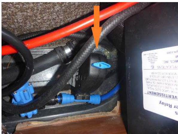
Alde frost control valve in operating position
