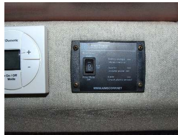
Inverter switch for optional 2500 watt inverter
