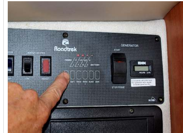
Tank status lights
