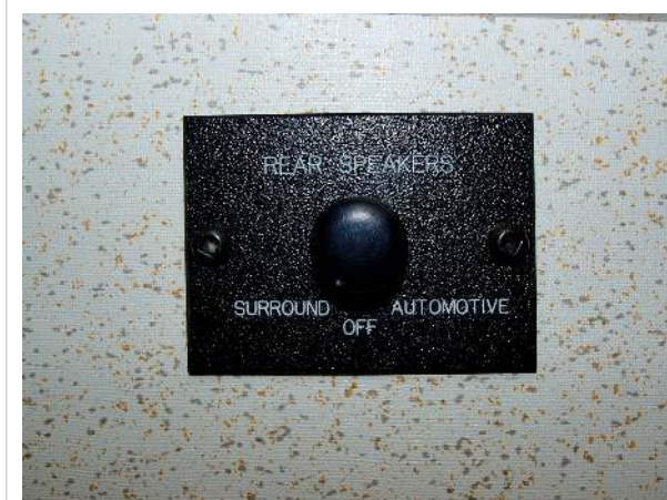
Rear speaker control switch
