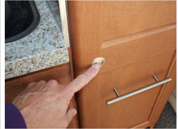
Locked pushbutton latch on cabinet door
