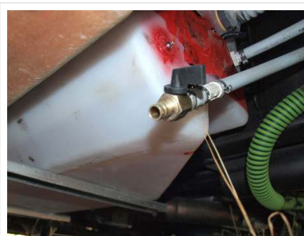
Exterior tank drain, under driver's door step
