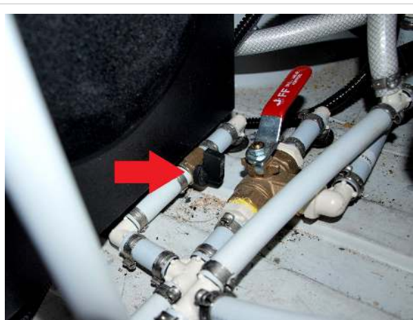
Valve connecting the interior and exterior tank, shown closed
