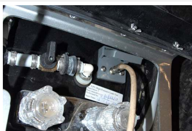
TV cable connected
