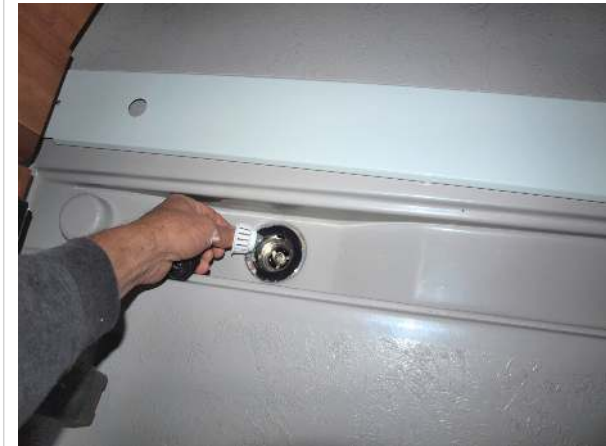
Aisle shower drain
