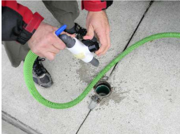
Open the waste water discharge hose valve
