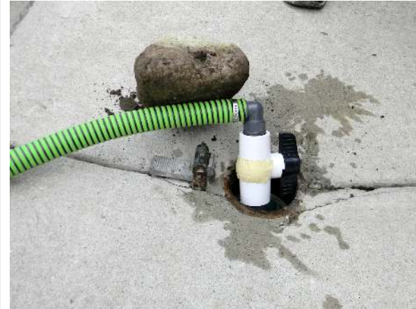
Weigh the hose down to prevent accidents
