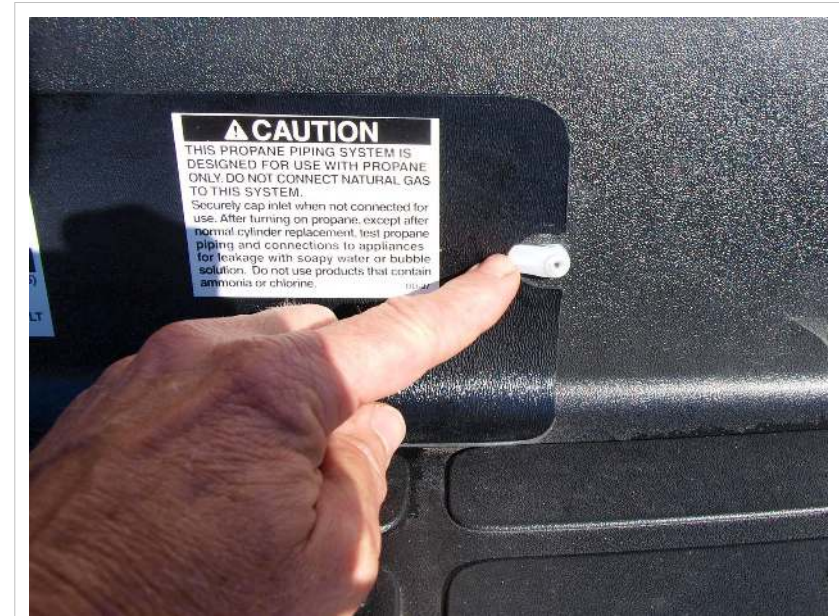
Propane access cover
