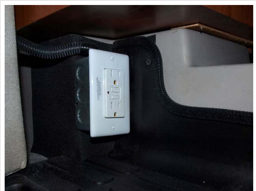
GFCI outlet under rear passenger side seat
