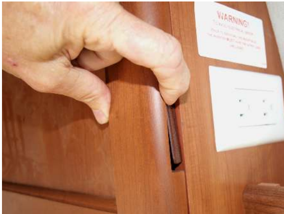
Hidden latch along edge of cabinet door
