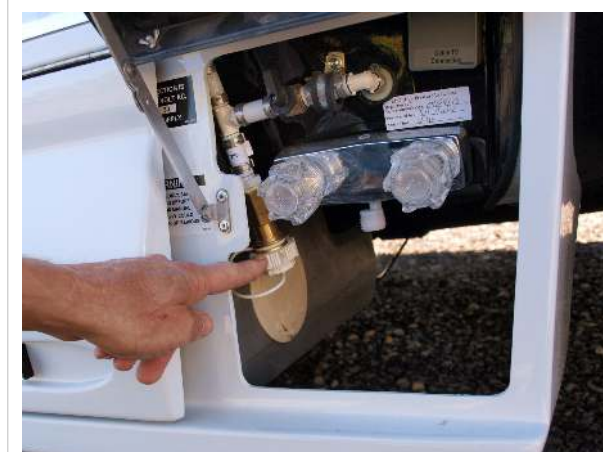
City water connection
