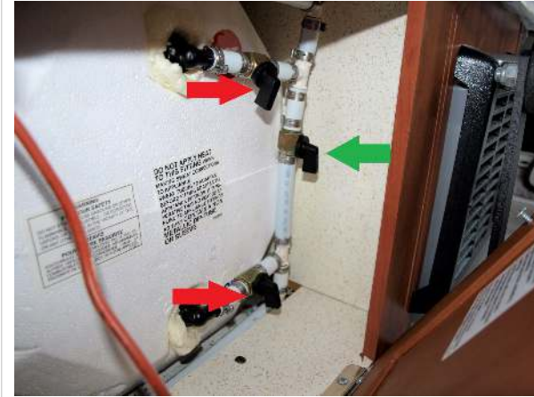
Water heater bypass valves in the bypass position. In the bypass position, all handles are vertical
