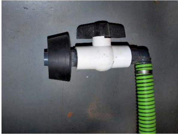
Rubber doughnut installed on nozzle
