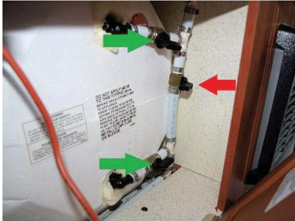
Water heater bypass valves in the open position. In the open position, all handles are horizontal
