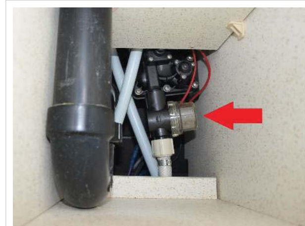
Water pump filter
