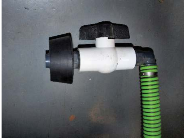
Rubber doughnut installed on nozzle
