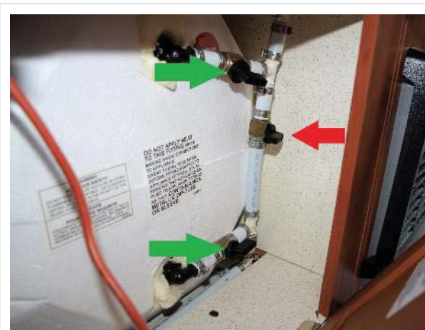
Water heater bypass in normal position - green arrow means valve is open; red means shut
