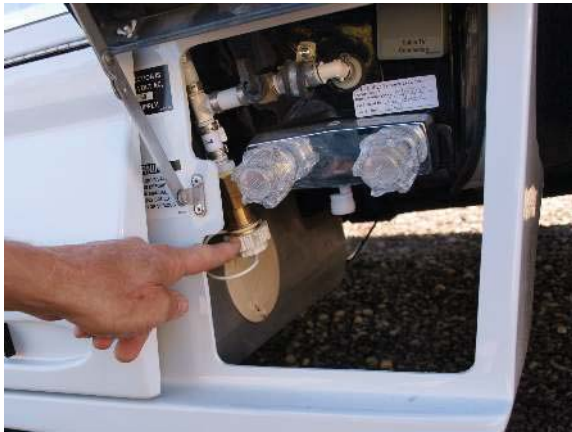
City water fill location
