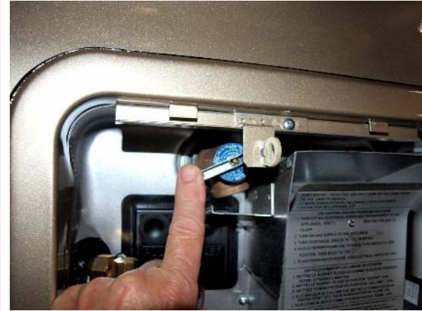
Water heater pressure relief valve
