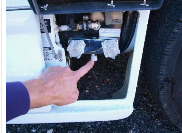
Driver's side rear access door
