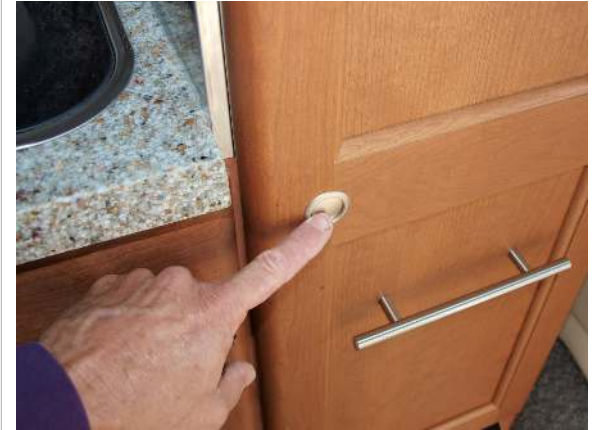
Locked pushbutton latch on cabinet door
