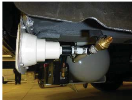
Drain by the fresh water fill in the rear
