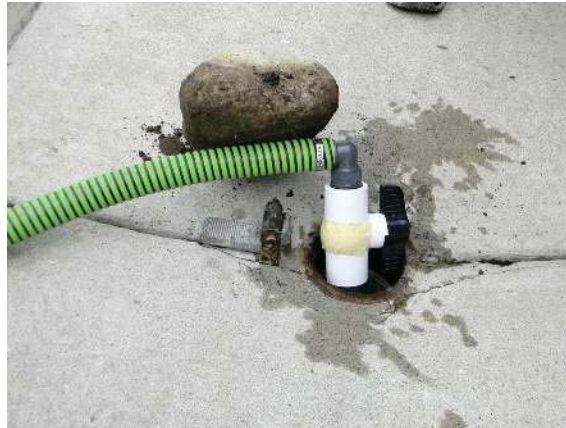
Use a rock or other weight to hold hose down
