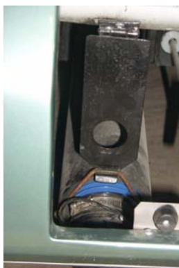
Picture G-P8: Sewage hose being supported by the carrier and support spring
