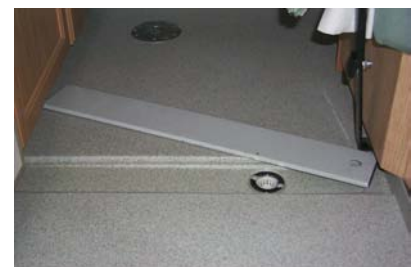
Picture B-P24: Floor drain, remove floor drain cover using the access holes provided in the cover.
