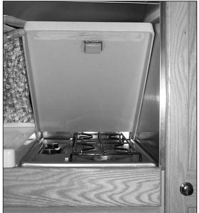
Picture B-P33: Lifting stove counter top.
