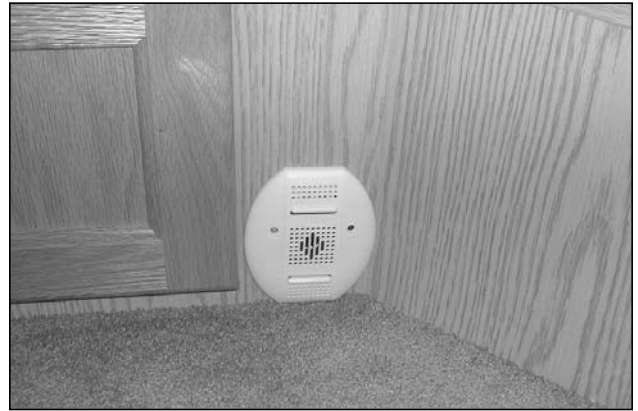
Picture F-P1: Propane leak detector.
