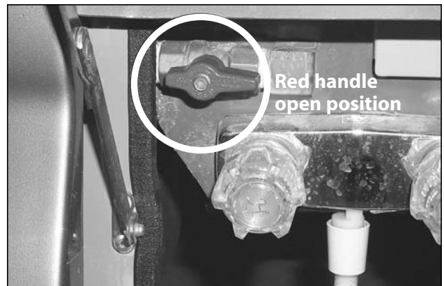
Picture G-P4: Open position of the city water tank fill valve.
