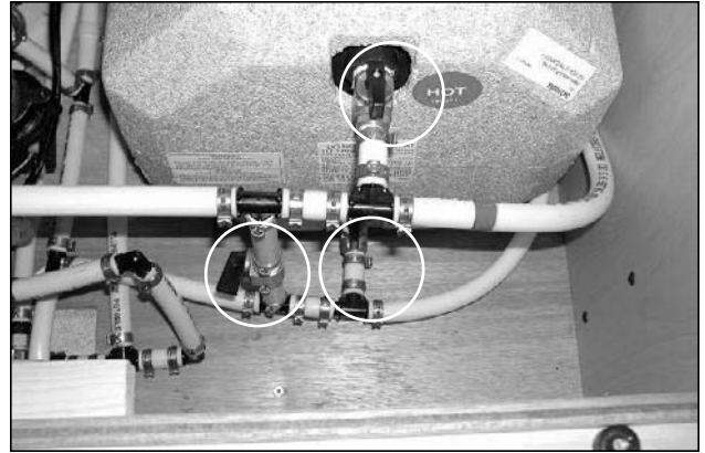
Picture G-P14: Summer mode valve positions.
