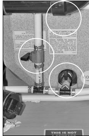
Picture G-P3: Summer mode valve positions.
