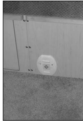
Picture F-P1: Propane leak detector, (Popular model).
