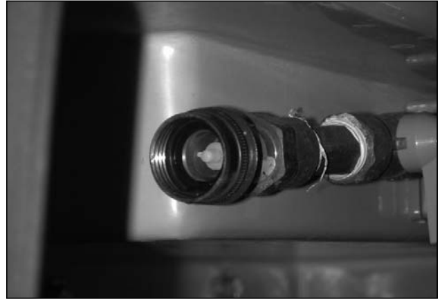
Picture G-P0: City water fill check valve.
