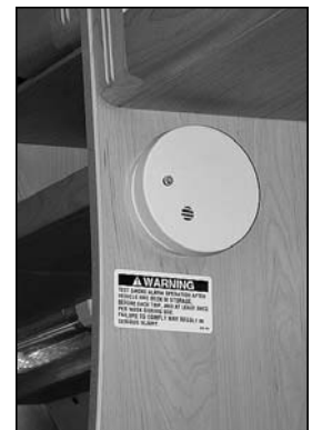
Picture F-P3A: Smoke detector, (Versatile model).
